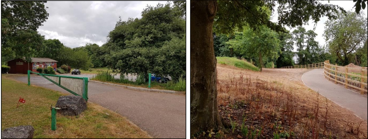
Existing infrastructure at Northbrook Approach
